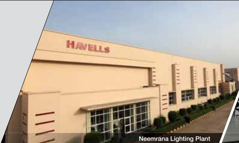
Neemrana Lighting Plant
